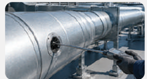
Duct Air Velocity
